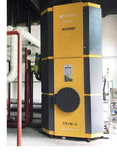
equipment, saving on capital expenditures. Also, in the case of using Electric Boiler, they eliminate the need for a stepdown transformer.
